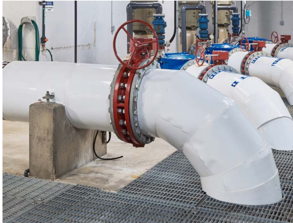
Figure 39: Wastewater Treatment Plant
