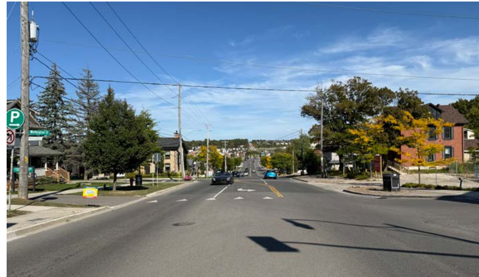
Figure 12: Broadway East (looking east towards Highway 10) from Wellington St.
