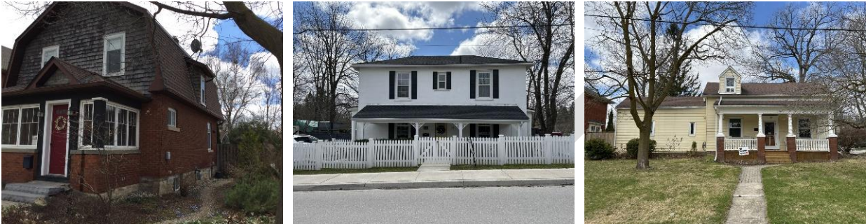
Photo 8 Examples of wood shingles (left), stucco (centre), and vinyl siding (right) in the HCD
