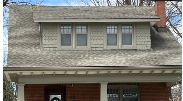
Photo 10 Examples of decorative shingling in the HCD including in a gable peak (left) and on a shed dormer (right)
