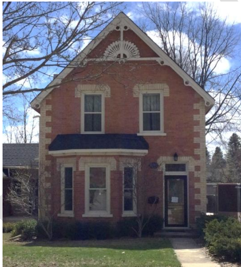
Photo 13 Examples of appropriate replacement windows in the HCD including the retention of existing openings and architectural elements
