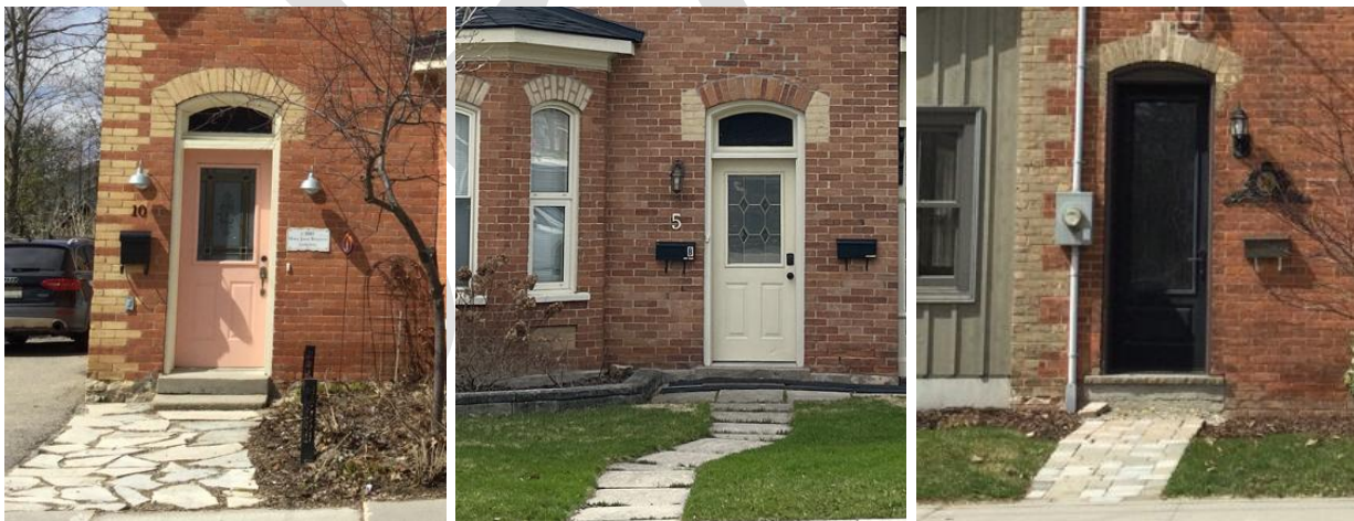
Photo 15 Examples of appropriate replacement doors in the HCD with retained original openings and architectural features
