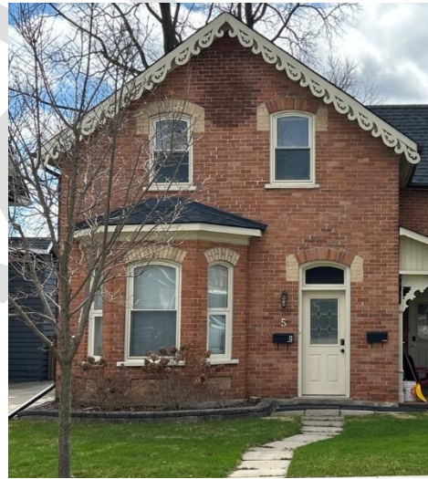
Photo 13 Examples of appropriate replacement windows in the HCD including the retention of existing openings and architectural elements
