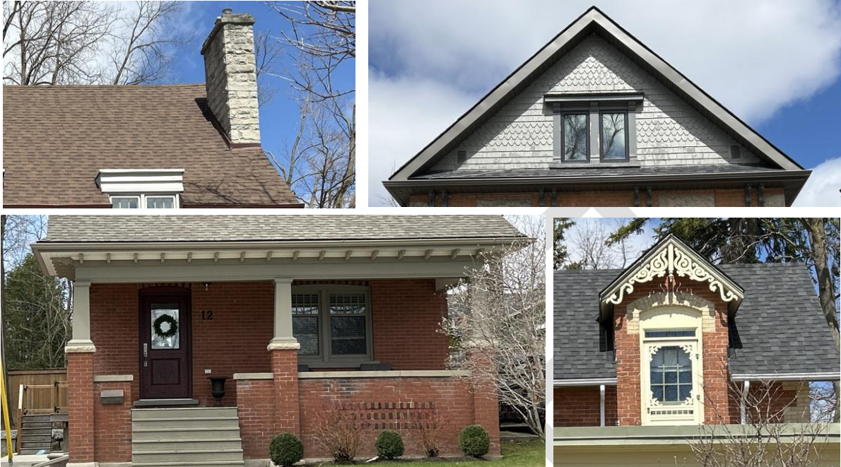
Photo 3 Examples of character-defining roof features in the HCD from top left to bottom right including stone chimney, gable, wide eaves with brackets, and dormer (See Appendix C for Architectural Terminology)
