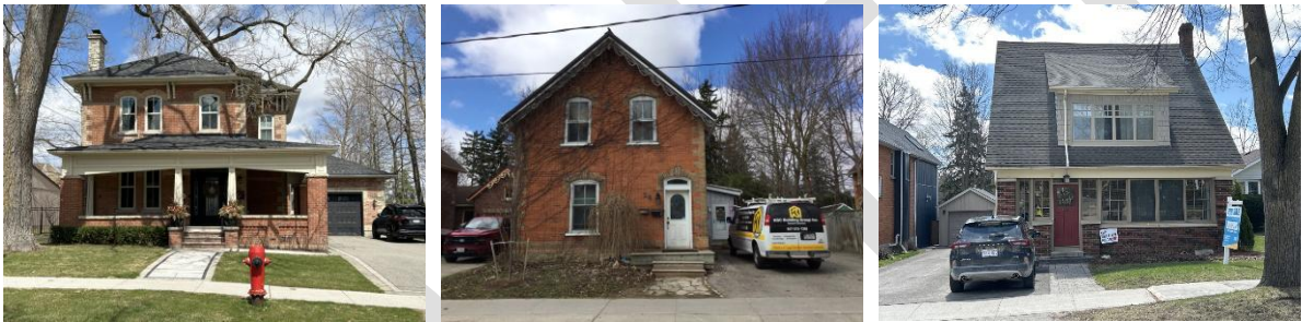
Photo 1 Low, medium, to high pitch roof examples on contributing properties, including hip (left) and gable roof (centre and right) types
