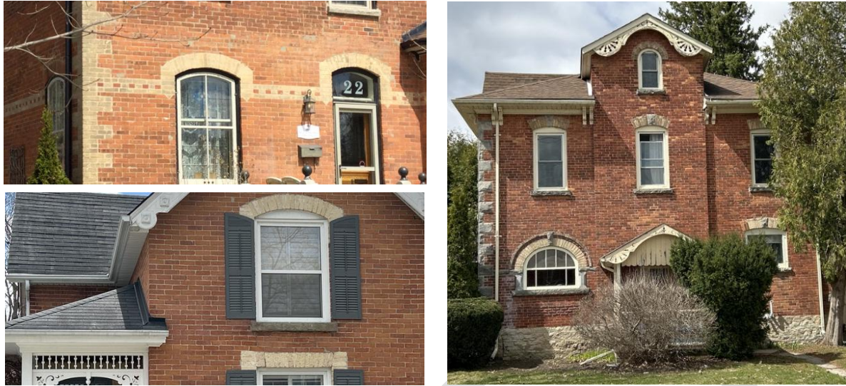
Photo 7 Examples of decorative brick and stone in the HCD including voussoirs, quoins, horizontal banding, arches (See Appendix C for Architectural Terminology)
