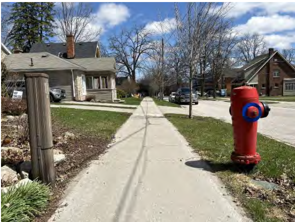
Photo 21 Concrete Sidewalk on York Street, Looking East
