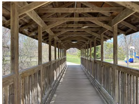
Photo 32 Covered Bridge, Looking North
