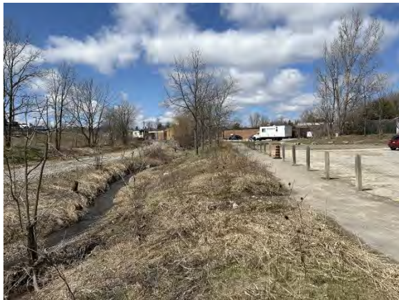
Photo 34 Multi-Use Path, Looking Northwest
