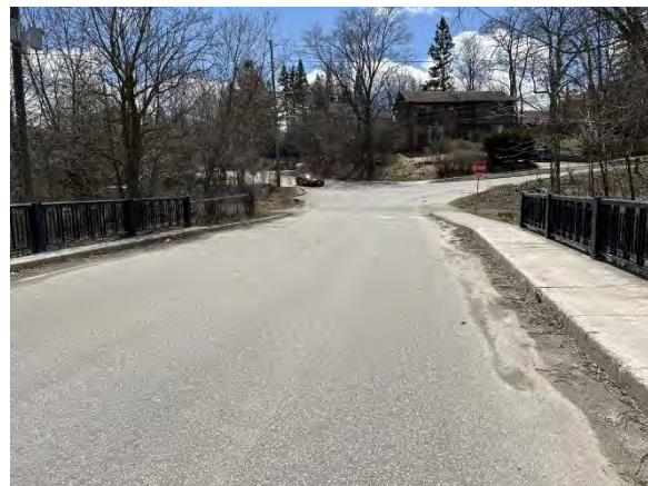
Photo 14 Bridge Across Mill Creek at Bythia Street, Looking South
