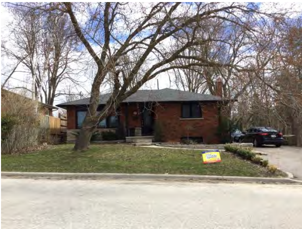
Photo 11 27 Bythia Street, Example of the Ranch Style
