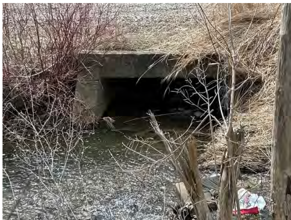
Photo 36 Culvert, Looking South
