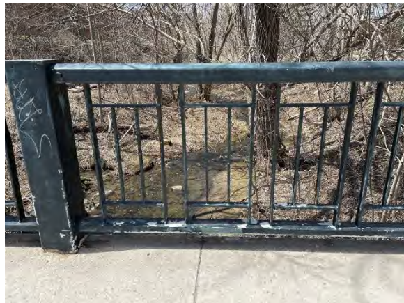
Photo 40 View of Mill Creek Through Bridge Railing on Bythia Street, Looking West
