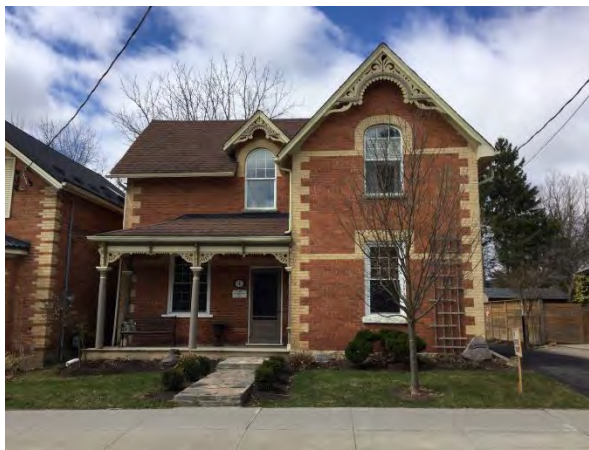
Photo 2 8 Bythia Street, Example of the Gothic Revival Style
