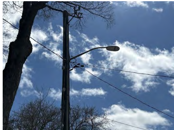
Photo 22 Streetlight Affixed to Utility Pole, Looking North
