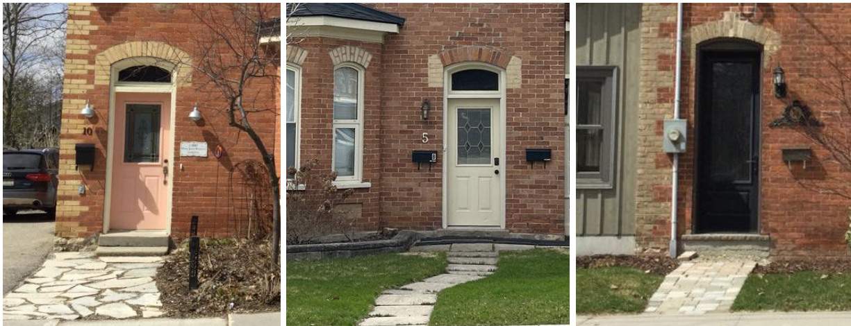
Photo 15 Examples of appropriate replacement doors in the HCD with retained original openings and architectural features
