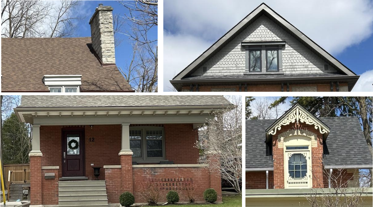
Photo 3 Examples of character-defining roof features in the HCD from top left to bottom right including stone chimney, gable, wide eaves with brackets, and dormer (See Appendix C for Architectural Terminology)
