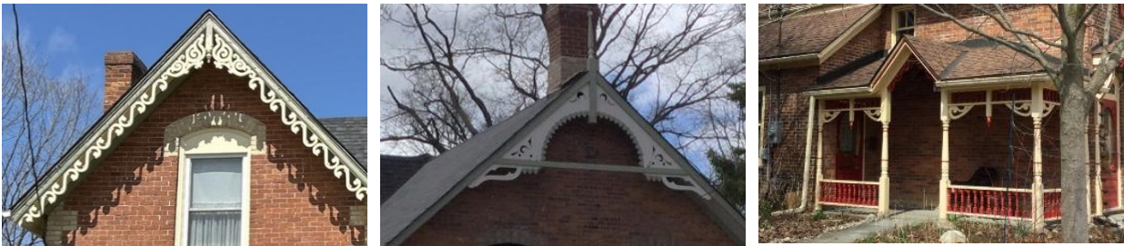
Photo 9 Examples of woodwork in the HCD including bargeboard (left and centre), window surrounds (left), and porch detailing (right)
