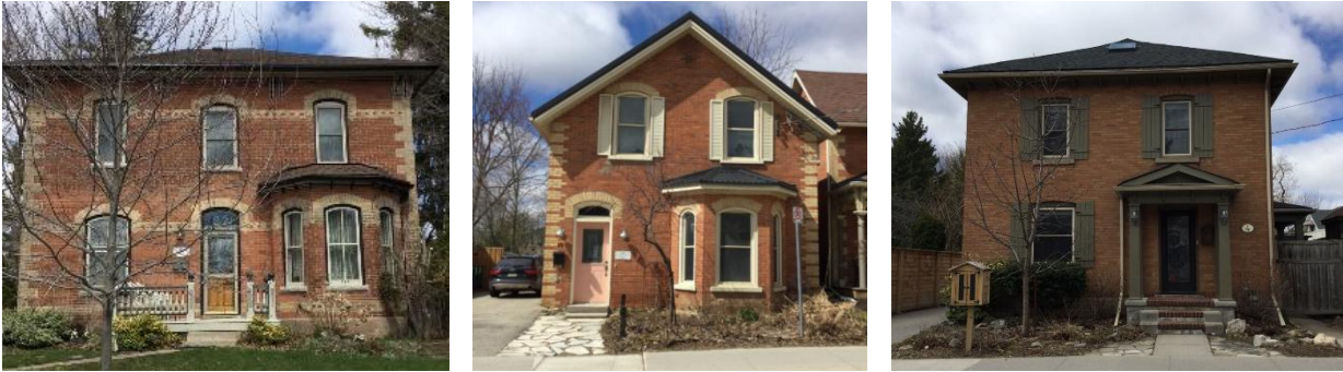
Photo 4 Examples of retained historic façade patterns including a three-bay front façade with central entrance (left), and two-bay front façades with off-set entrances (centre and right)
