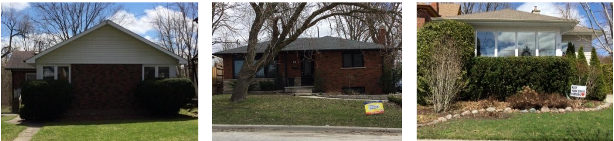
Photo 2 Example of low-pitched gable (left) and hip roof (centre and right) types on non-contributing properties in the HCD
